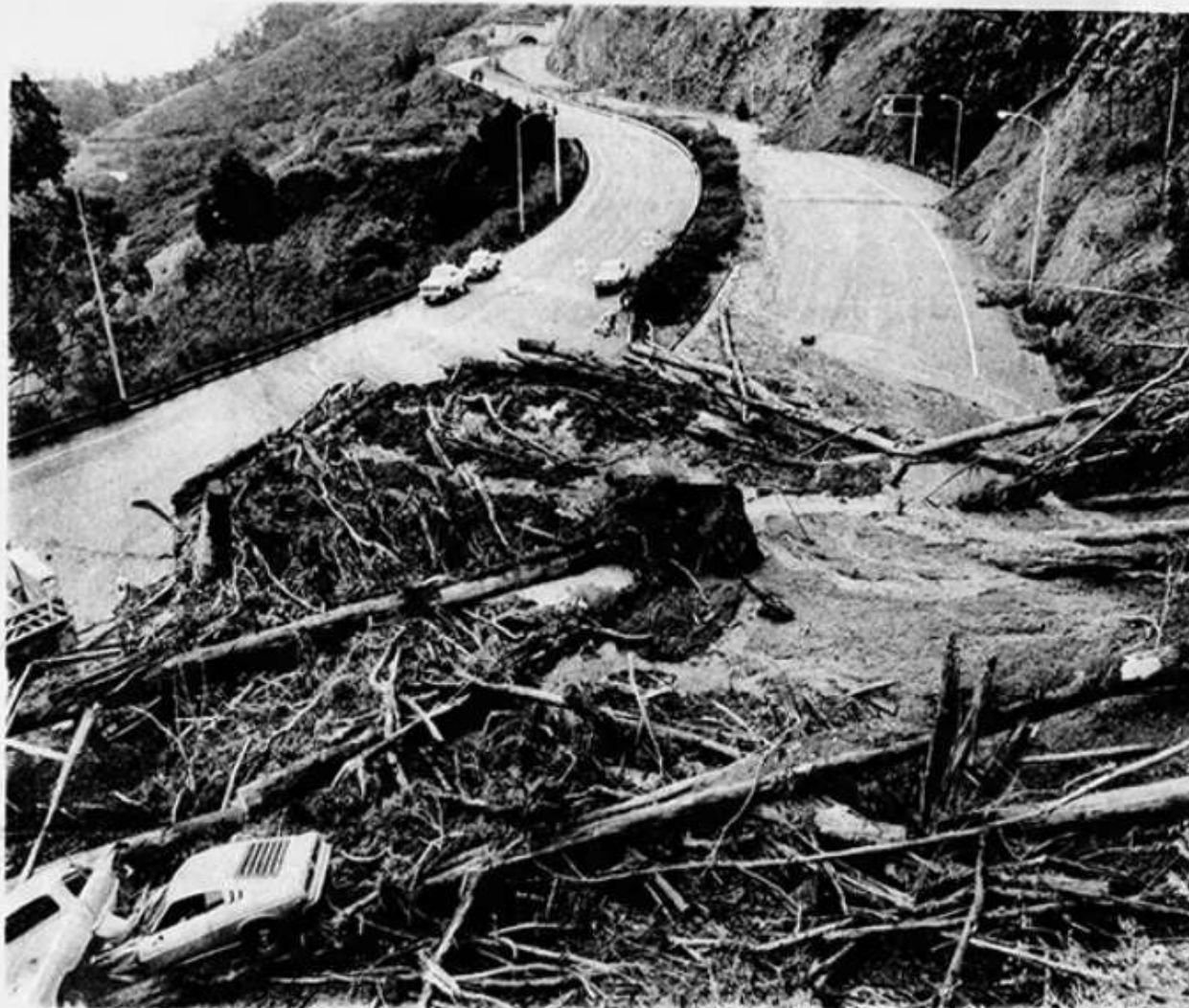
Mudslides at Waldo Grade have closed Highway 101 and further threaten to erode the soil underneath the roadway and collapse the tunnel
